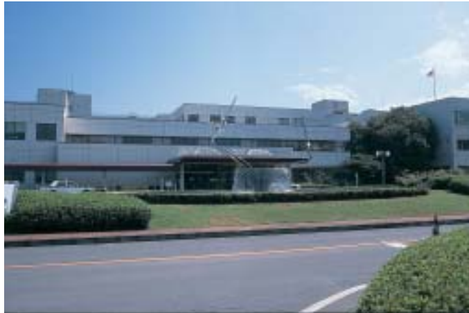
附属病院正面 Main Entrance to University Hospital
